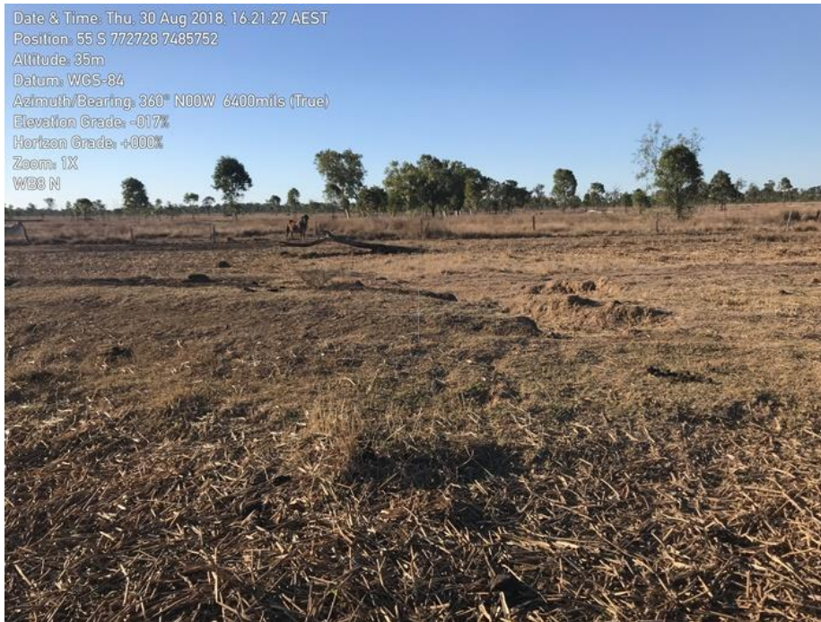
Photo looking north from WB8a showing some erosion but no channel
